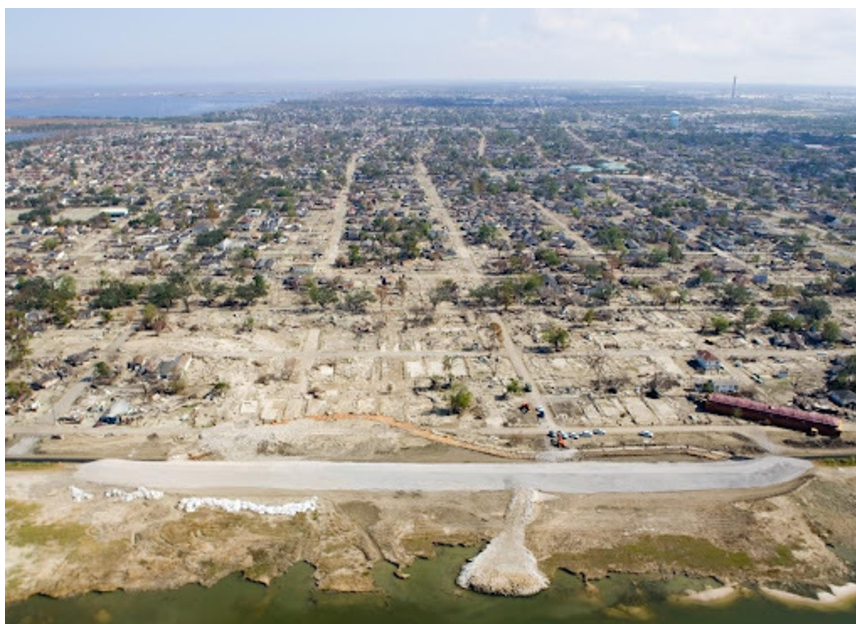
November 8, 2005: View of the damage from the breach of the Industrial Canal to the Lower Ninth Ward after the water receded. Photo courtesy of George Long, from his book Katrina Days: Life in New Orleans after Hurricane Katrina . 1
